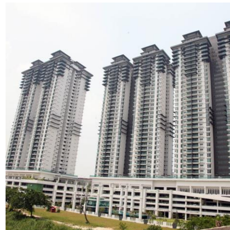
Kiara Residence 2 Bukit Jalil, KL - 720 units Condominium Developer: Kiara Residence Properties Main Contractor: Wong Brothers Building Construction S/B
