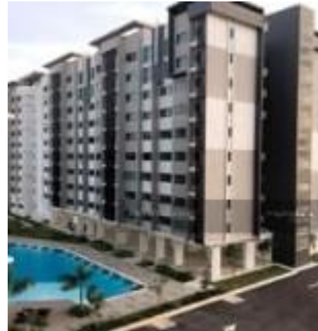
Suria Rafflexsia Setia Alam - 360 units Medium cost apartment Developer: Sunsuria Berhad Main Contractor: Permai Ihsan Sdn Bhd
